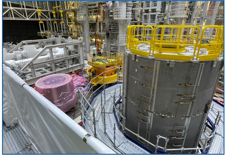
US ITER is delivering the “heart of ITER,” the superconducting central solenoid magnet. The first two magnet modules are stacked for assembly. Photo: US ITER
